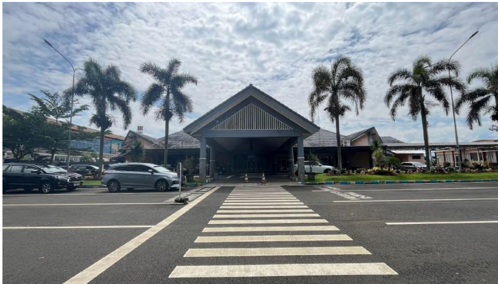
Figure 2. Abdulrachman Saleh Airport Arrival Terminal, 2025 (source: Personal Documentation, 2025)
