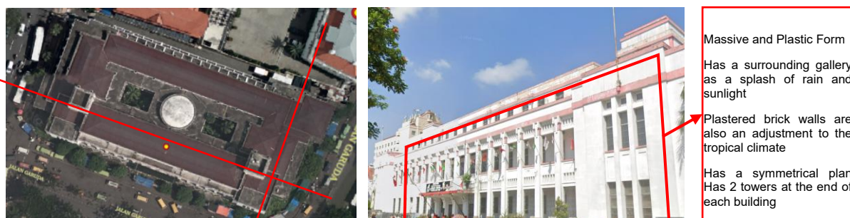
Figure 5: The Massive and Plastic Form of the Internatio Building Source: https://petaperuntukan.dprkpp.web.id/ and author
