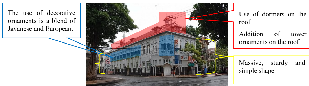
Figure 9: Image of BNI Bank Building KCP 46 Jembatan Merah
