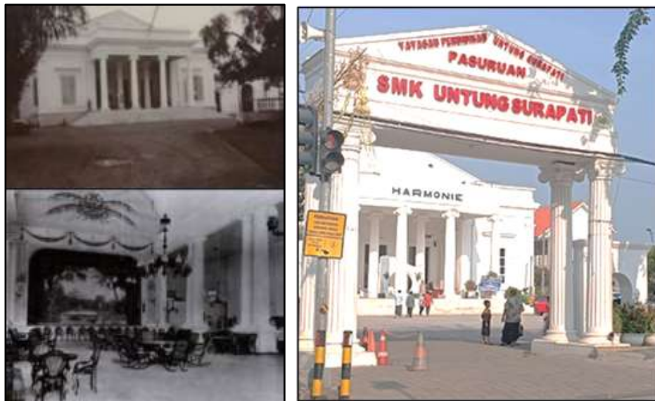
Figure 6. Harmonie Societie Building then and now.
