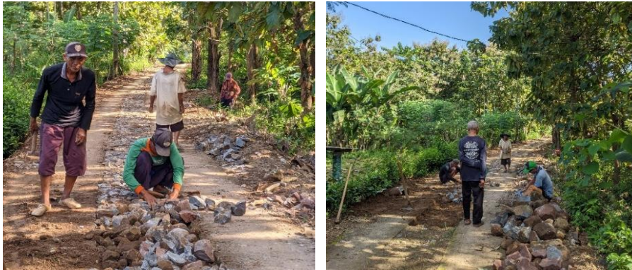
Figure 4. Installation of the macestone
