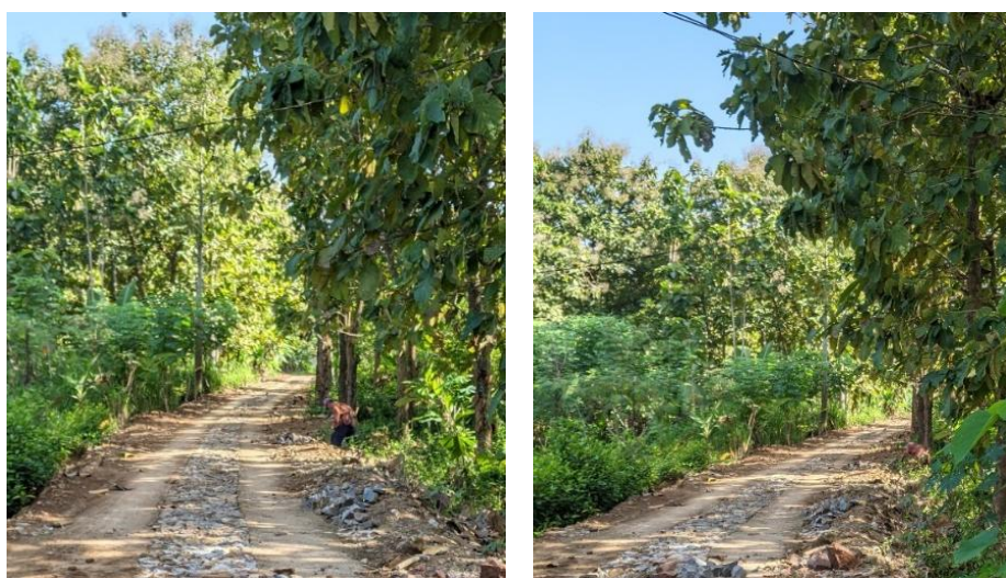
Figure 6. Finished Makadam Road
