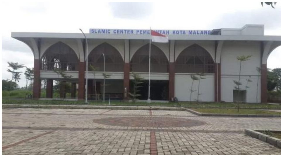
Figure 2. Building facade Source: (Google, 2025)
