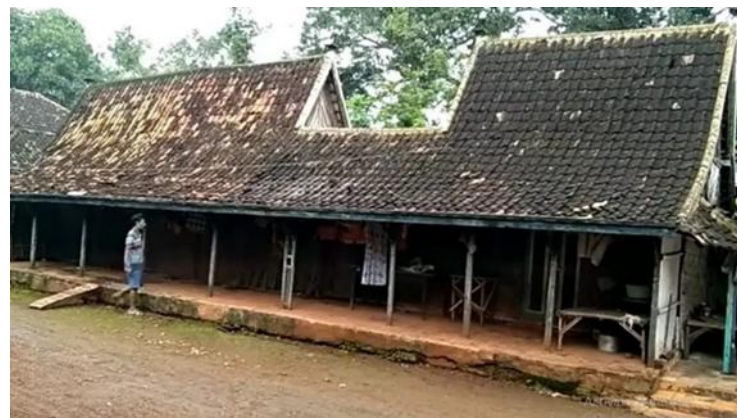
Figure 5. A traditional Madurese house with a Trompèsan-style roof (Source: Epi Abdul Haris)
