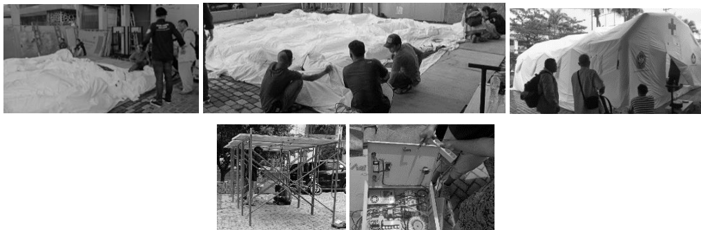
Figure 2. Installation of Inflatable Tents and Solar Power Plant
