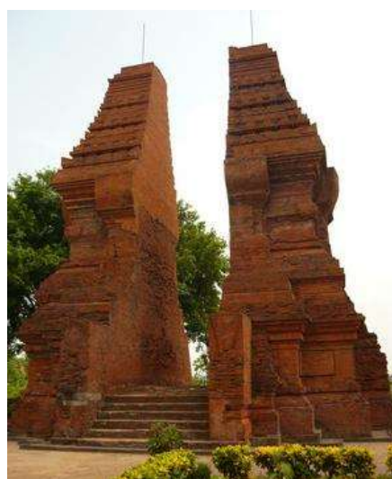
Figure 3. Wringin Lawang Temple, Trowulan District, Mojokerto Regency. Showing the shape of the gate of the Candi Bentar type, which is the same as the relief at Candi Jago, Malang Regency
