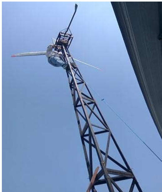
Fig.6. Installation of HAWT on pole.
