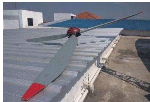
Fig.4. Blade is ready to install
