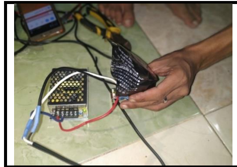
Fig 4. Photocell Testing in Dark Conditions
