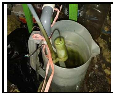
Fig. 6. Water Pump Testing
