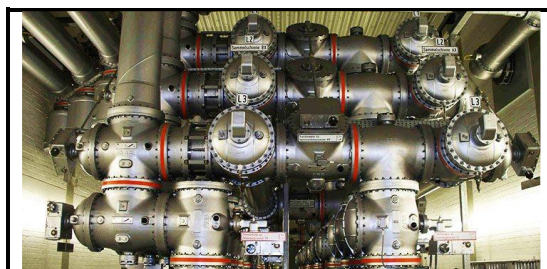
Fig 1. Compartment for Desiccant Trial
