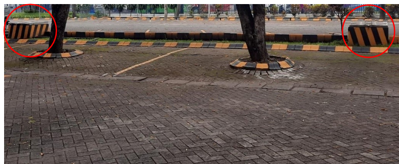
Gambar 4. Dua Manhole Ground Tank.
