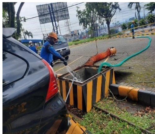
Gambar 10. Proses Pengurasan Air.
