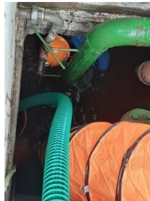
Gambar 9 Proses Cleaning Groundtank
