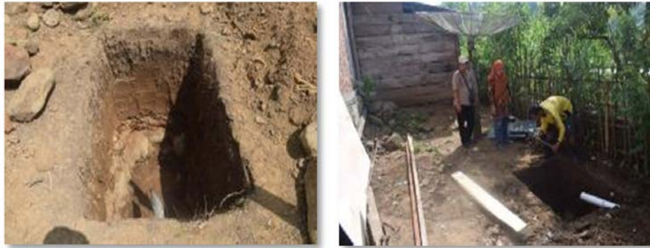
Figure 5. Preparing septic tank
