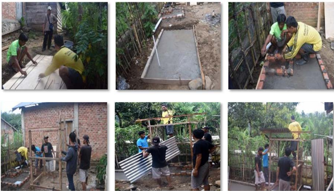
Figure 6. Assistance in building foundations, roof frames, and walls
