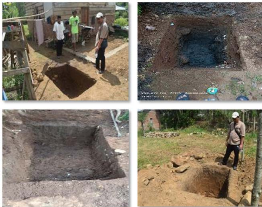
Figure 2. The septic tank holes in (a) Dusun 1; (b) Dusun 2; (c) Dusun 3; and (d) Dusun 4 of Air Pesi Village
