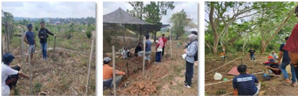
Figure 1. Survey of water treatment plant construction sites
