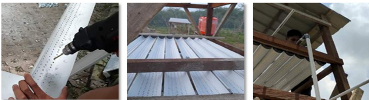
Figure 3. Aeration tray and pipe installation process
