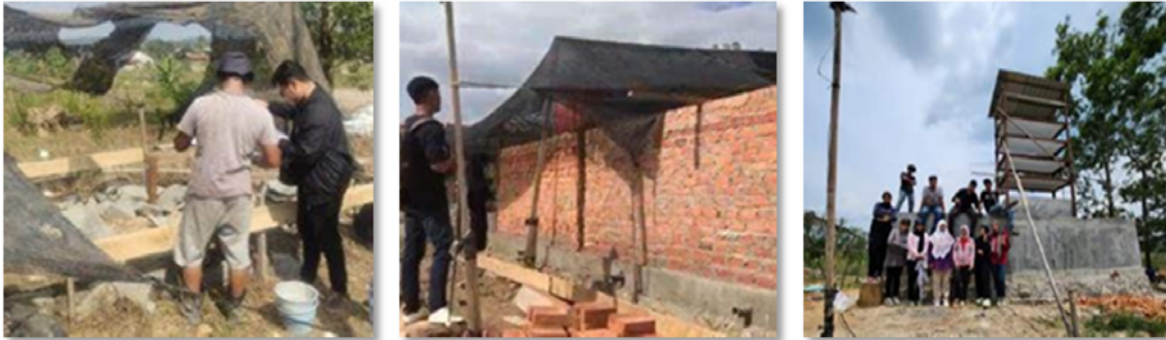
Figure 2. Water treatment plant construction process
