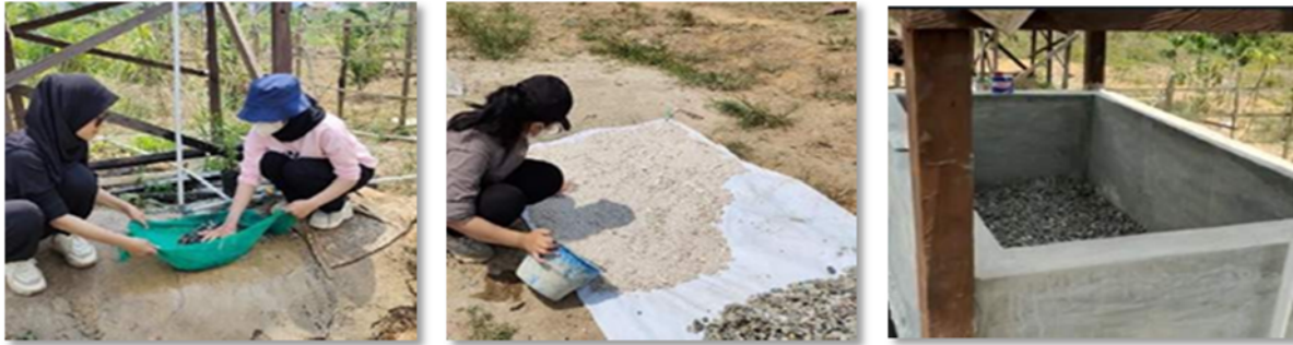
Figure 4. Media cleaning and filling process
