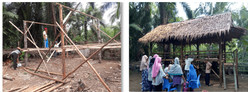
Figure 9. The working lodges
