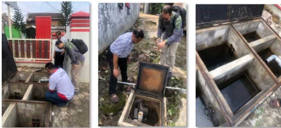
Figure 7. Installation of anti-bacterial water filter system
