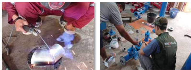
Figure 5. Assembly process of the hydrum pump
