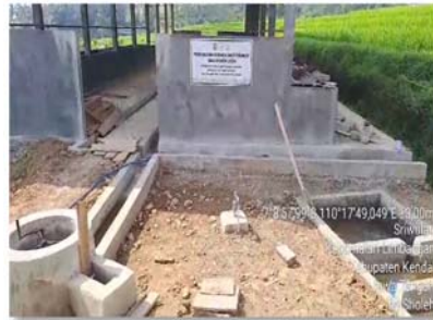
Figure 5. Location of the biodigester
