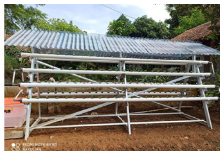
Figure 2. Installation of DFT vertical hydroponic system
