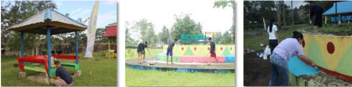
Figure 6. Repainting bordname and gazebos
