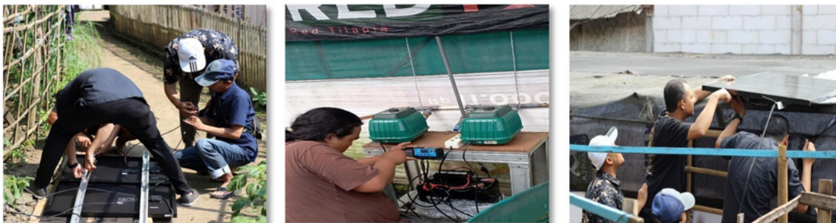
Figure 3. Solar panel system installation
