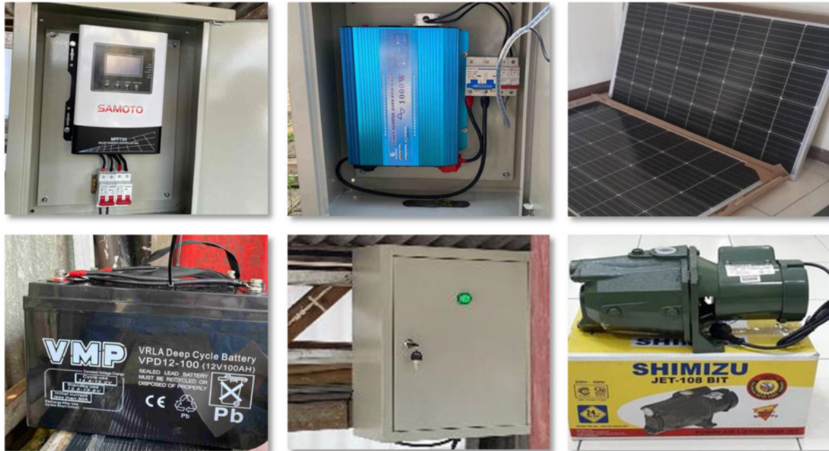
Figure 4. Tools on solar panel installation for water pumping machine: Solar Charge Controller (SCC) 60A, inverter 1000W, monocrystalline solar panel, panel box, accu 12V/100 A, and water pump
