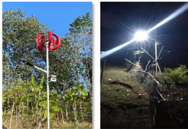
Figure 11. (a) Complete design of VAWT-based PJU, (b) Condition of VAWT-based Public Street Lighting at Night
