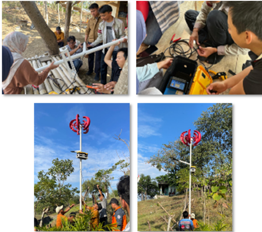
Figure 9. (a) Installation of PJU cables to poles; (b) Installation of power transmission systems; (c) Installation of VAWT and PJU; (d) Validation of system performance of installed PJU
