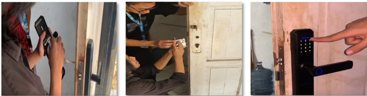
Figure 5. Smart door lock main system installation process
