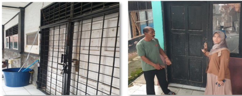
Figure 3. Smart door lock system installation location
