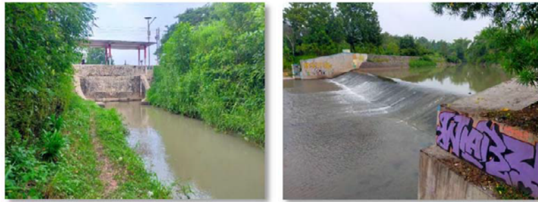
Figure 1. Location of potential water resources in Bekacak
