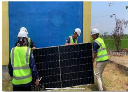
Figure 4. The process of installing the solar panels
