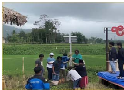
Figure 8. Installation of real-time land monitoring equipment in Jenggawah Village
