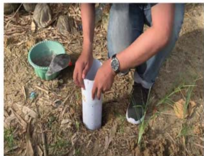
Figure 3. How to install biopore infiltration hole pipe into the ground
