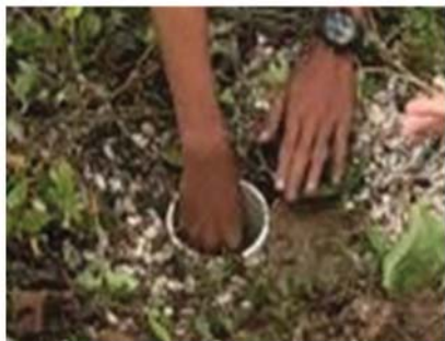
Figure 3. How to install biopore infiltration hole pipe into the ground
