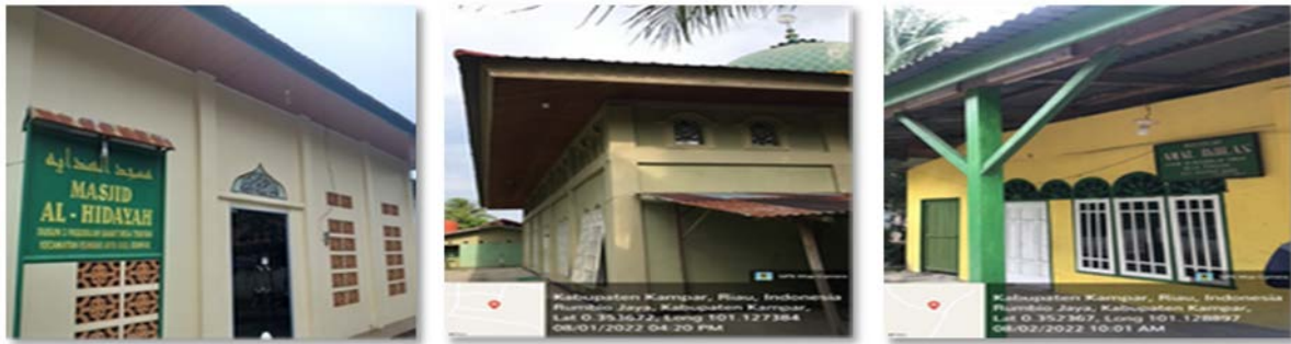
Figure 11. Worship facilities survey results
