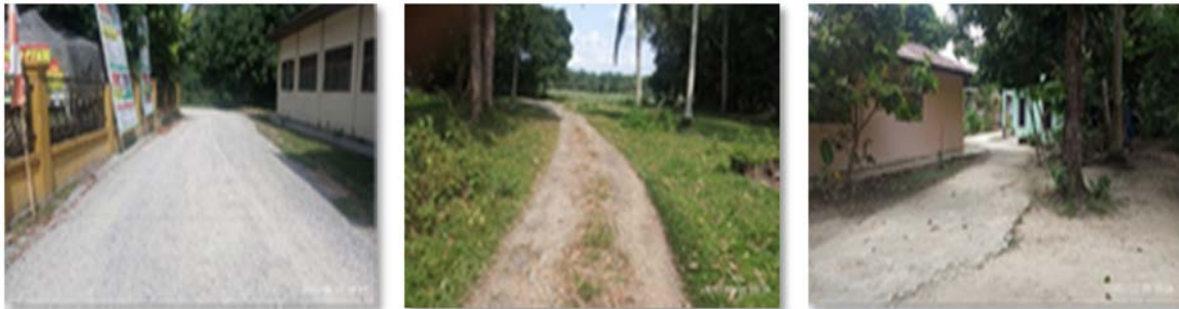
Figure 8. Road infrastructure survey results: (a) Asphalt pavement; (b) Soil pavement; (c) Cement pavement
