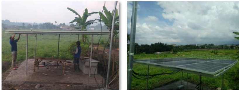
Figure 7. Construction of solar panel support poles
