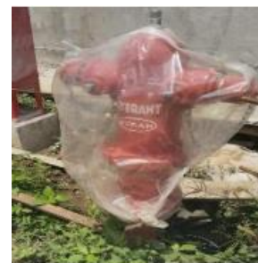
Figure 2.5 Pillar hydrant
