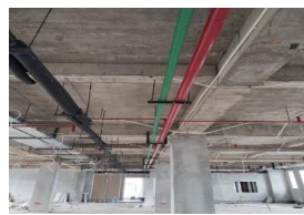
Figure 2.2.a. Pump piping installation, b. Building/hydrant
