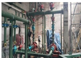
Figure 2.2.a. Pump piping installation, b. Building/hydrant
