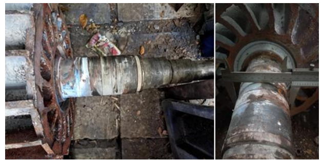
Figure 5. Visual Inspection and Dimensional Measurement
