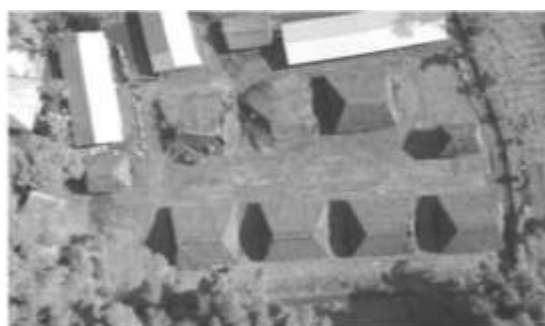
Figure 7. The condition of the Traditional House of Sembalun Village during an Earthquake of seven on the Richter scale (Source: Susilo et al., 2019)
