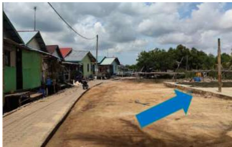
Figure 6. Grounds with concrete pavement in Tiangwangkang
