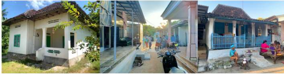
Figure 2. Elevating the floor levels of the residential houses of the Bugis-Makassar community
