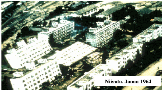
Gambar 3.5: Earthquake Effects - Liquefaction (Lisa Wald, USGS Pasadena) http://profile.usgs.gov/professional/mypage.php?name=lisa
