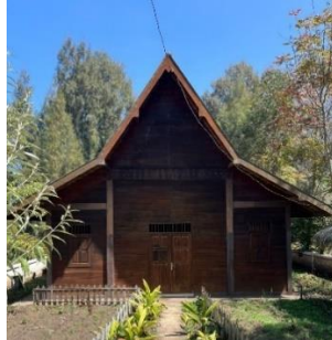
Figure 4. Traditional House of the Tengger Tribe Source: Personal documentation (Prasetya, 2024)
