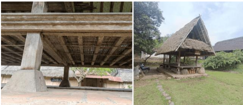
Figure 12. The Tenganan house construction Source: Author, 2025
