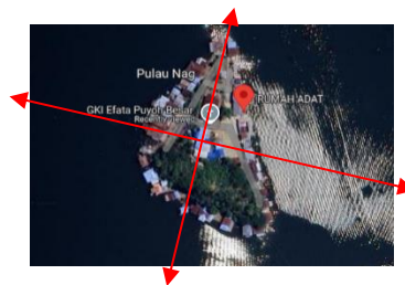
Figure 5. Layout of the GKI Efata Building from Kampung Putali Puyo Besar (Source: Google Maps, 2024)
