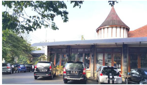
Figure 3. Building Jl. Arjuno no 36 west side (2015)
