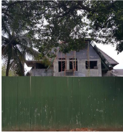
Figure 20. The building of Jl. Rinjani no 17 (2015)
