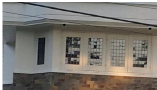
Figure 18. Window Elements on Second Floor (2015)
