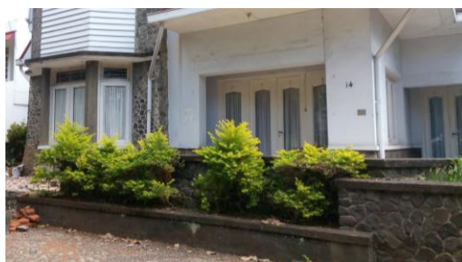
Figure 13. Wall and Openings Elements on the first floor (2015)
