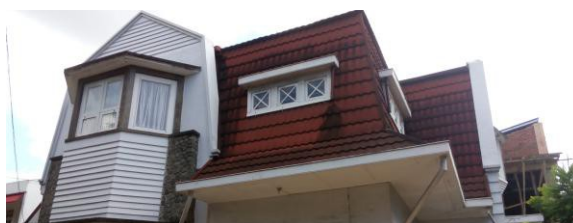
Figure 12. Roof, Wall and Building Openings on the second floor (2015)
