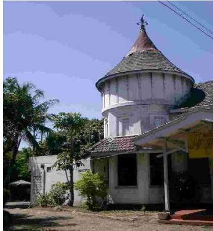
Figure 2. Building Jl. Arjuno no. 36 (2004) (Source: Antariksa, 2004)
