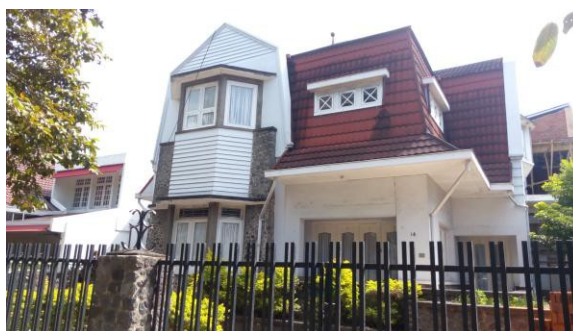
Figure 11. Building Jl. Tenes no 14 (2015)
