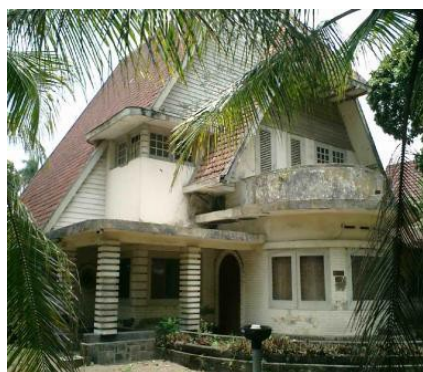
Figure 19. Building Jl. Rinjani no. 17 (2004) (Source: Antariksa, 2004)
