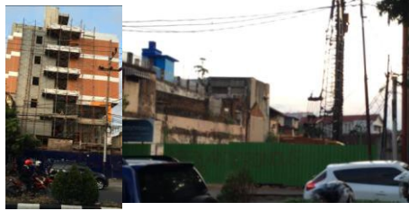
Figure 5. Demolition and construction of new buildings in Kayu Tangan
