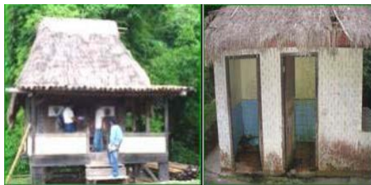
Figure 15. Police Station and Rest Room
