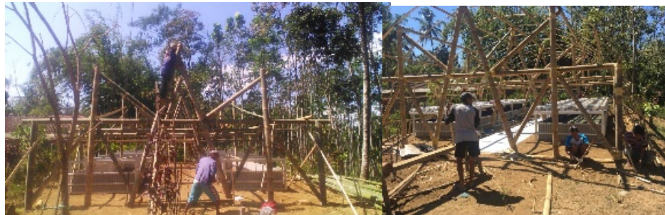
Figure 4. Construction of a Greenhouse (15 days)
