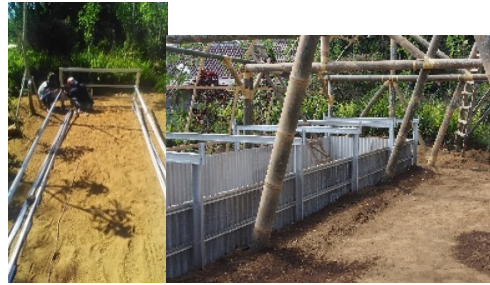
Figure 5. Hydroganic Installation (6 days)
