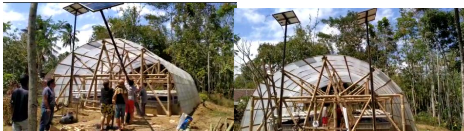
Figure 6: PLTS Installation (2 days)
