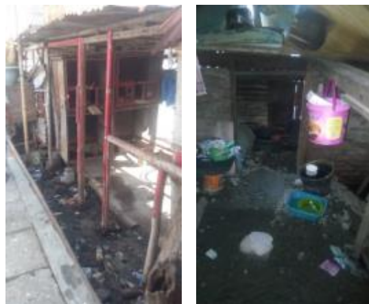
Figure6. Shows the overhead structures with different materials used for storage purposes. (Source: taken from the site 22 Oct 2019)
