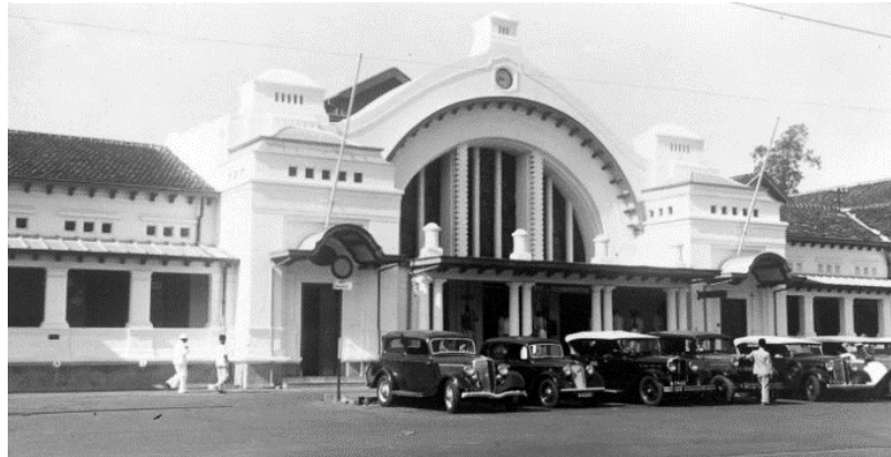
Figure 4. Photo of Filateli Building from the outside, taken in 1938.
