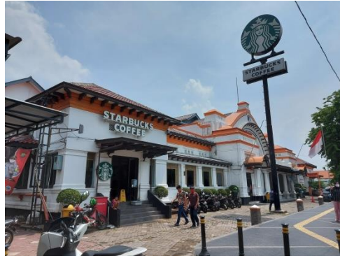
Figure 6. The exterior of Starbucks Filateli Building in 2020.
