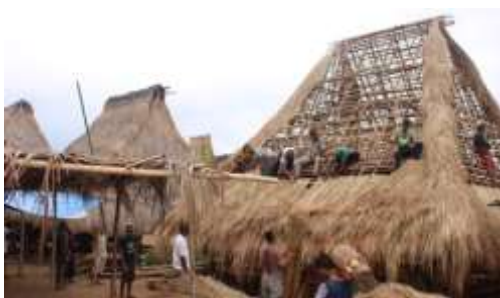
Figure 3 Rebuilding one of traditional house in Kampong Nggela
