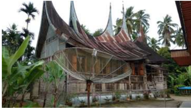
Figure 2. Gadang Jopang Manganti House, Munka, Limapuluh Kota, West Sumatra as the object of study (Source: author documentation)
