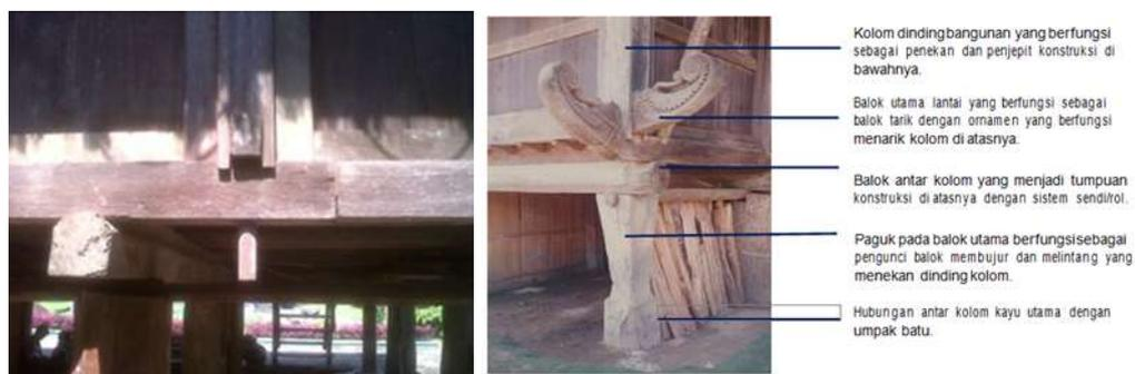
Figure 8 and 9. Support Systems, Pinch, Push and Pull Systems
